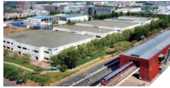
■ 北京第二工厂/The second factory 占地面积 / Total land area: 60,589m 2 建筑面积 / Total floor area: 40,222m 2
